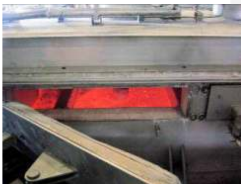
Figure 7 Reactor chamber of degassing system viewed with skim door open.
