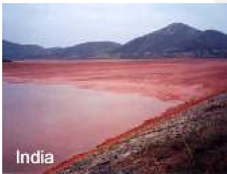
Fig.5. Lagoon type red mud disposal
